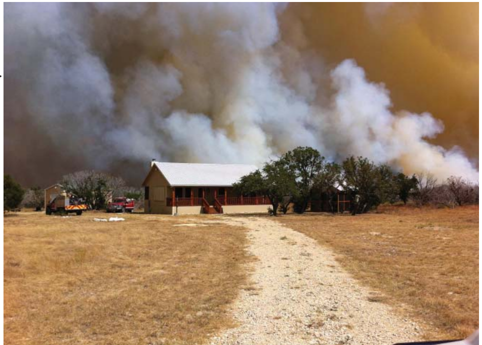
Even with minimal fuel to burn, wildfire can ignite homes and spread rapidly through combustible attachments.
